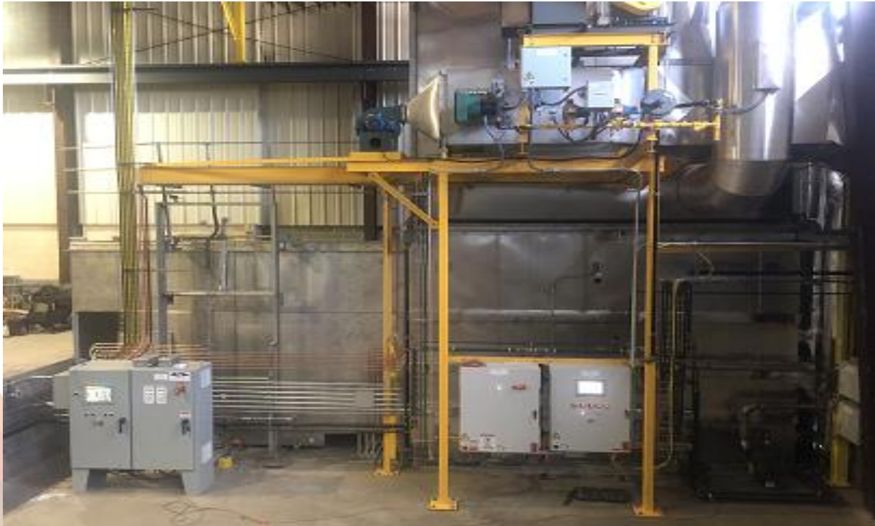
One of three Chem tanks at ProCurve Glass
