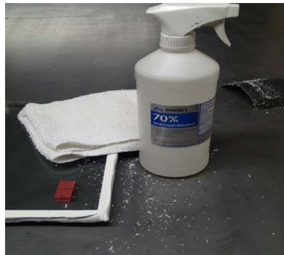
Image 2 – Applying IPA clean-wipe to abraded sealant surface
